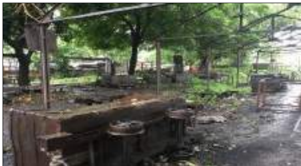
Before- Existing Structures (Pre-Dismantling)
