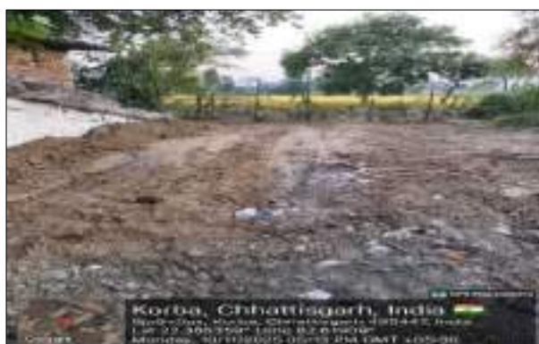
After- Sealed and Secured
