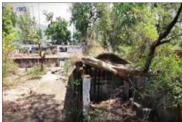
Before- Mine Entry Prior to Closure
