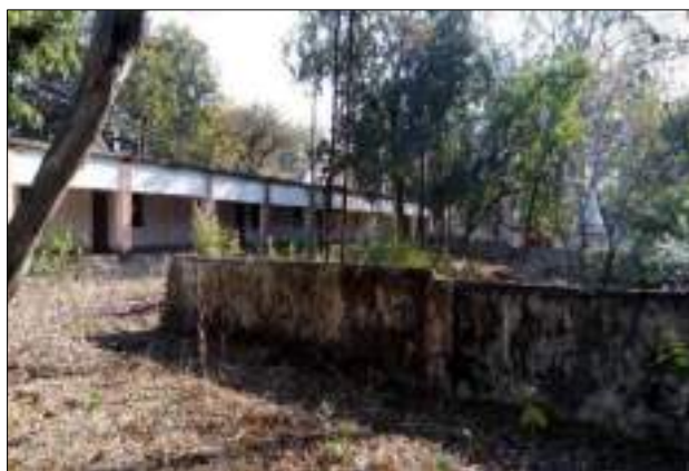
Before- Existing Infrastructure (Pre-Dismantling)
