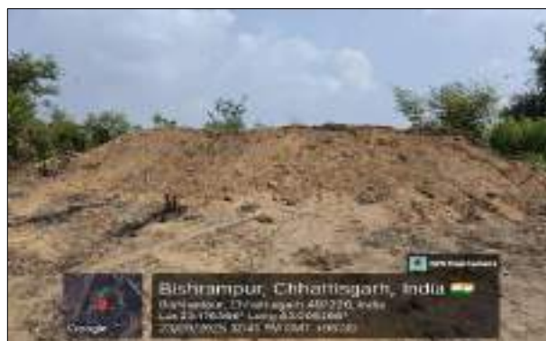
After- Entry Sealed with Concrete Fill and Stabilized with Soil Cover
