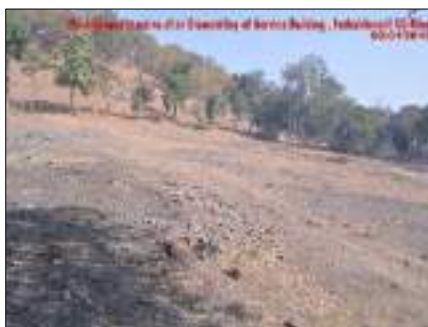
After-Site cleared & levelled for plantation
