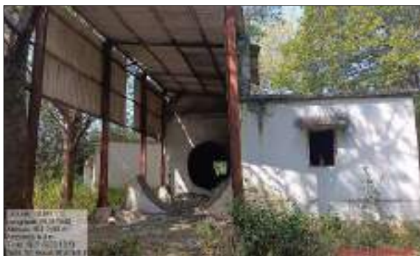
Before- Airshaft structure prior to dismantling
