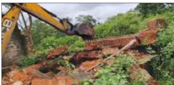
Before- Existing Structure (Fan Shaft)
