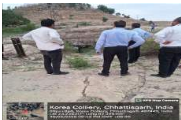
Before- Open Mine Entry (Pre-Closure)
