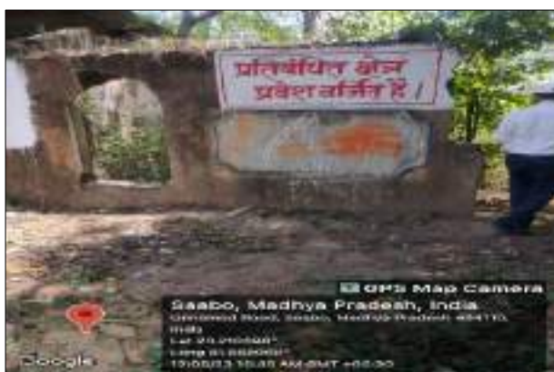
Before- Existing Structure (Pre-Dismantling)
