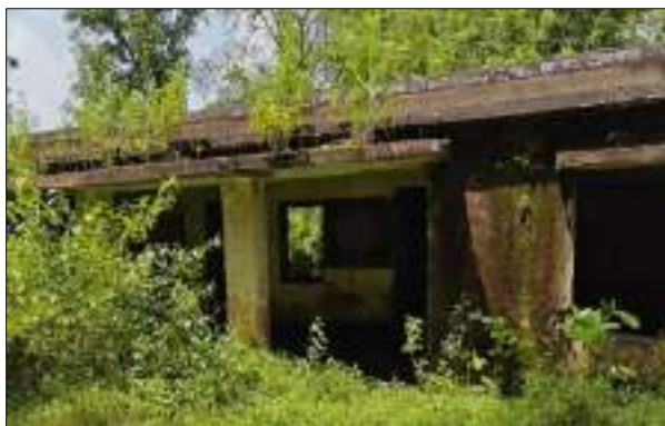
Before-Abandoned concrete structure
