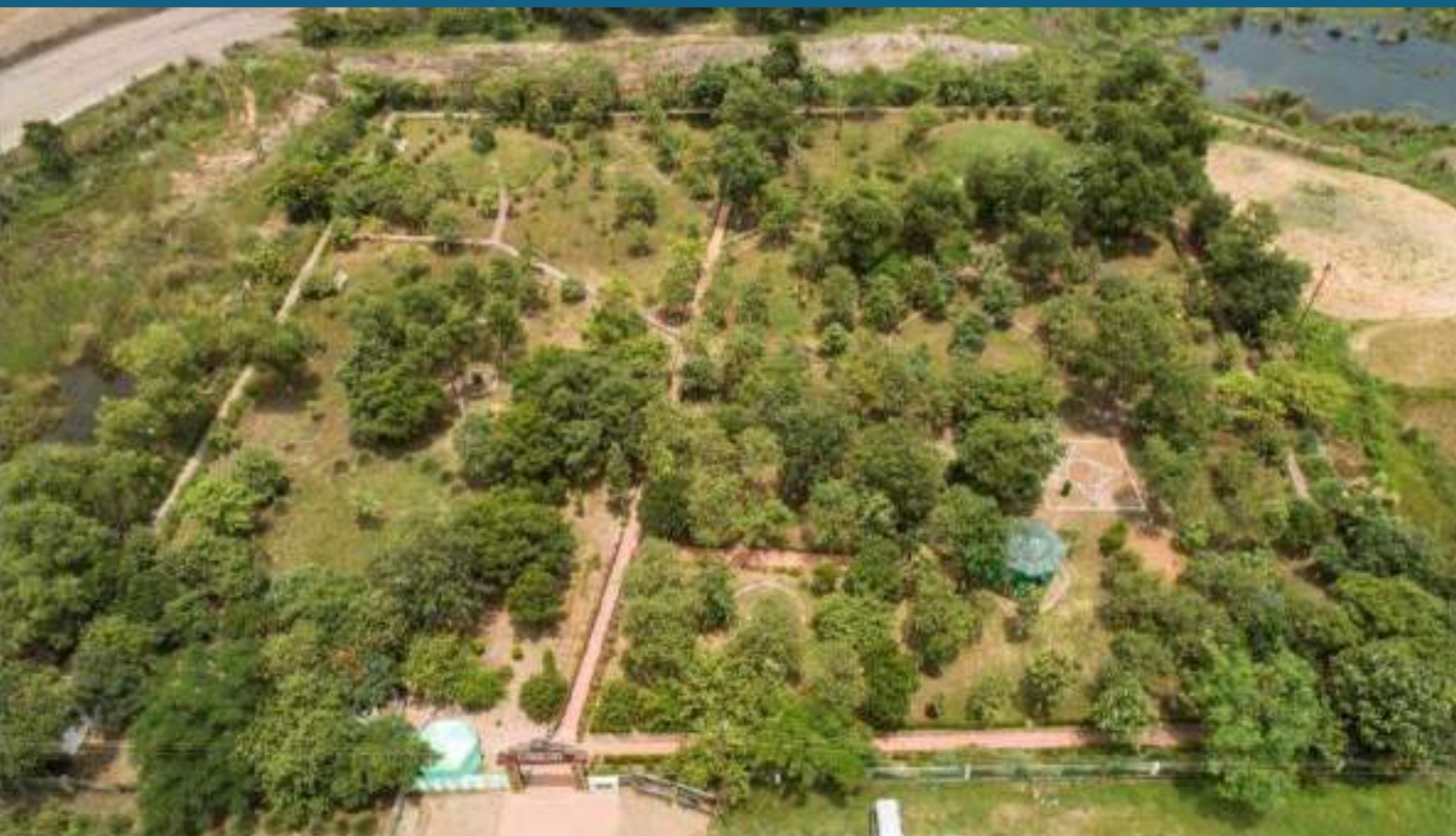
Aerial View- Eco Park Developed over backfilled area
