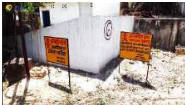
After- Secured and concrete sealed Incline
