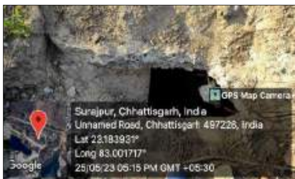
Before- Open Mine Entry (Pre-Closure)
