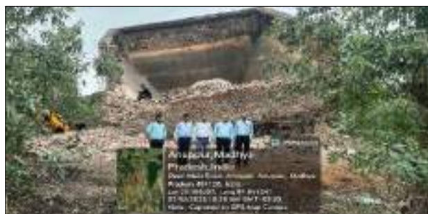
Before - Pre-Demolition Condition of Site
