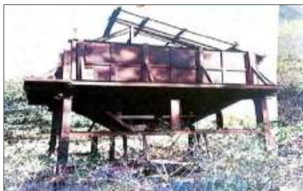
Before- Existing Structure (Pre-Dismantling)
