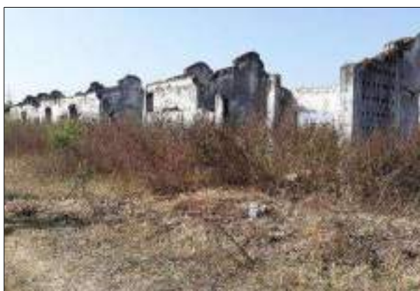
Before-Obsolete structure on site
