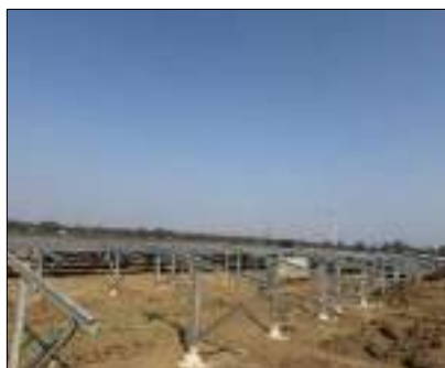
Solar Plant under installation
