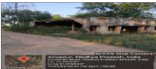
Before- Pre-Dismantling Condition
