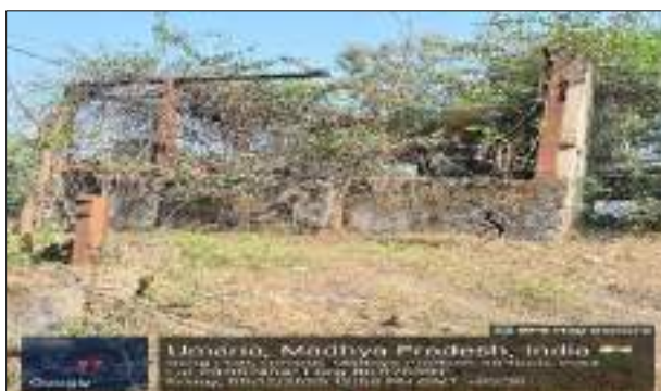
Before- Existing Structure (Pre-Dismantling)
