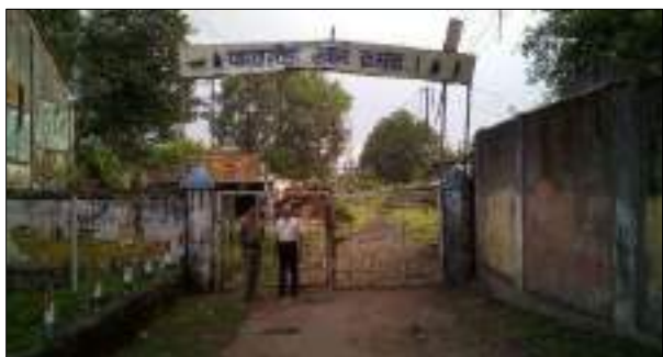
Before- Existing Mine Infrastructure
