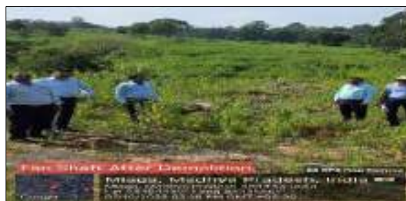
After- Cleared and Restored Site
