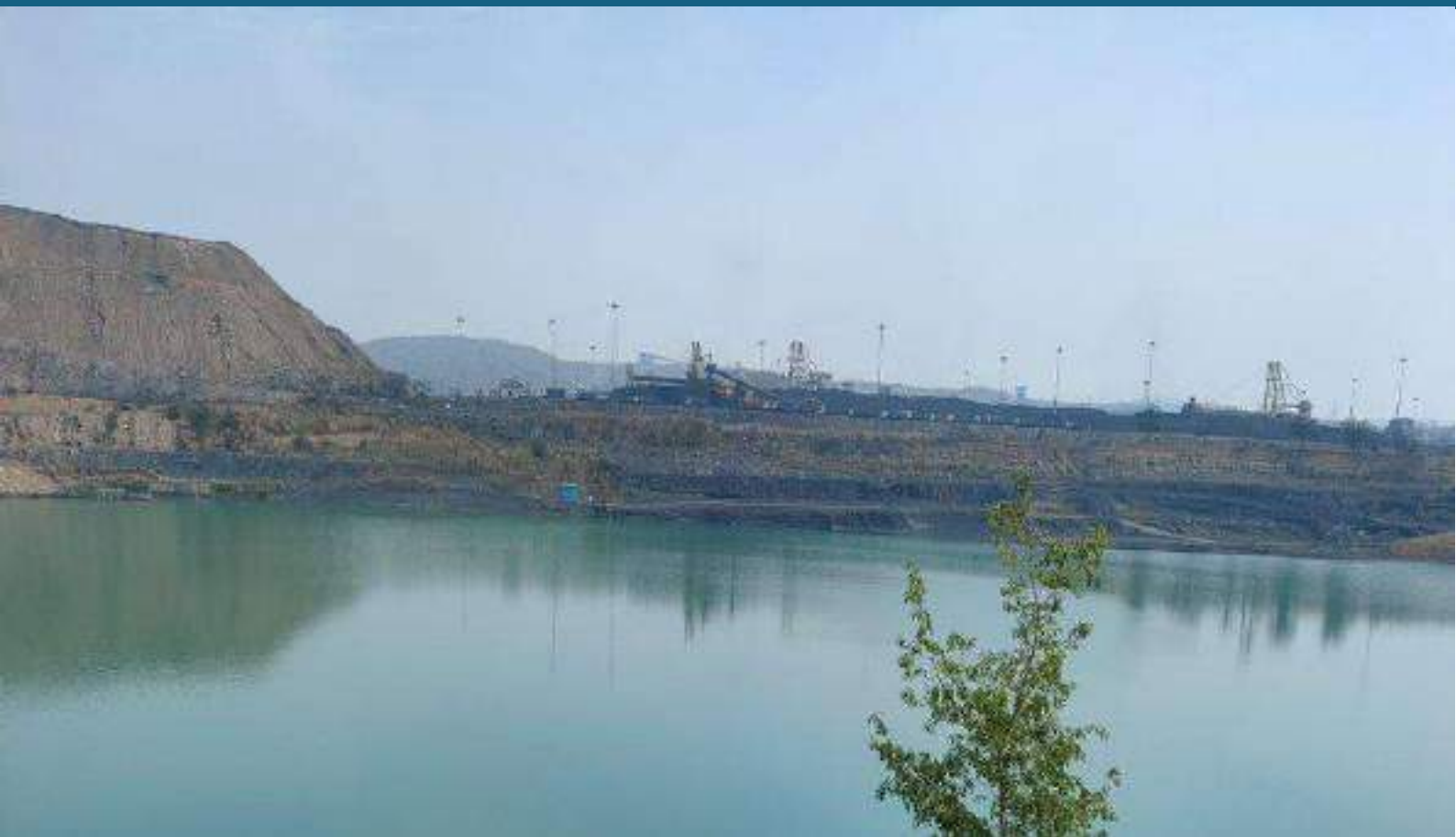
Storage of Approx. 23 Lakh m 3 Rainwater in Reclaimed Mine Area
