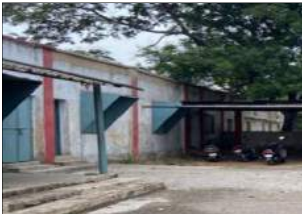
Before-Existing Building Structure
