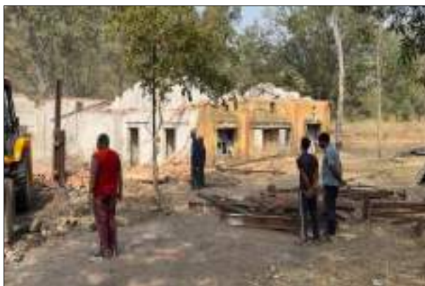
Before- Existing Structure (Pre-Dismantling)
