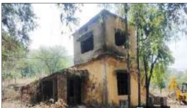
Before- Existing Structure (Pre-Dismantling)
