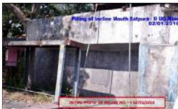
Before- Pre Closure Condition
