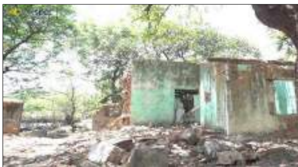
Before- Existing Structure (Pre-Dismantling)
