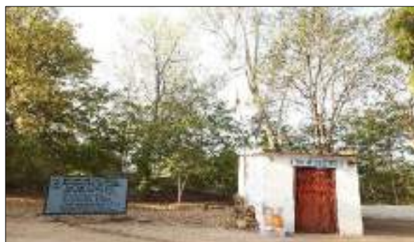
After-Incline entry sealed and secured
