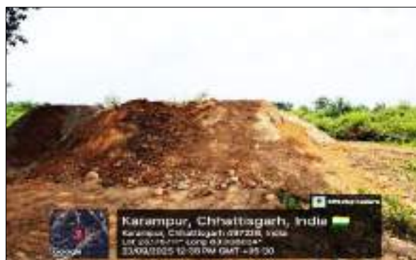
After- Sealed and Stabilized Entry
