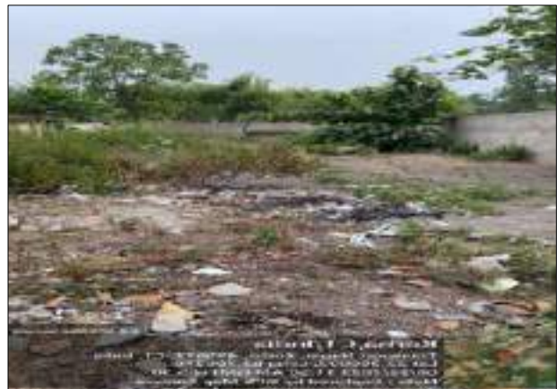
After- Site Cleared Following Demolition Activities
