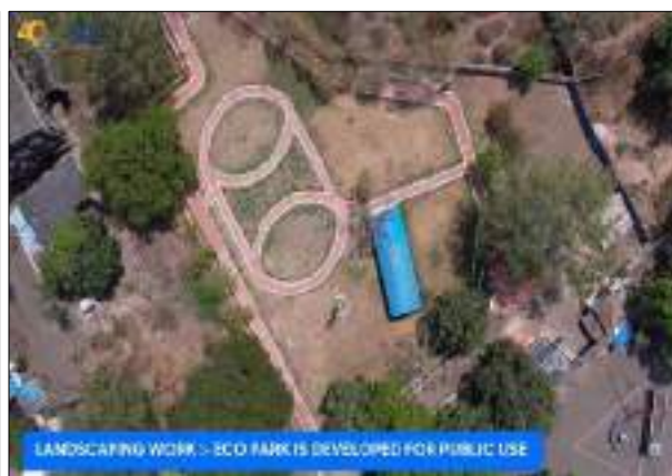
Aerial View- Development of Eco Park
