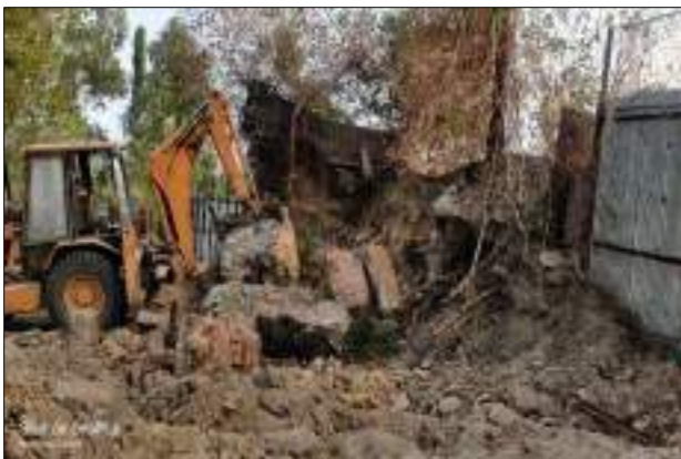
Before- Existing Structure (Pre-Dismantling)
