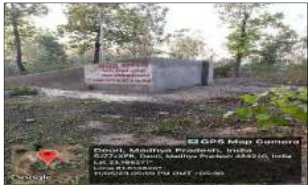
After-Sealed and secured
