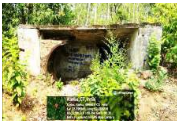
Before- Open Mine Entry (Pre-Sealing)
