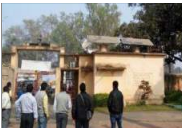
Before- Dismantling of Existing Structures
