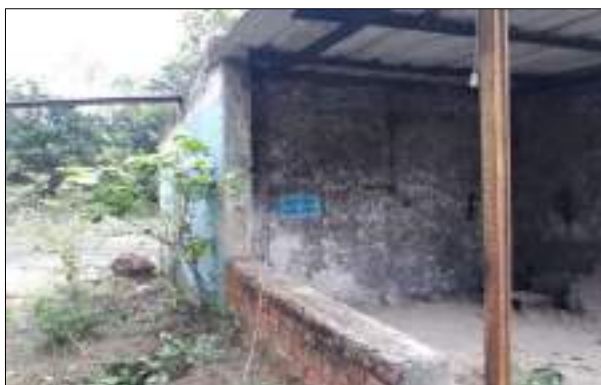
Before- Pre-Dismantling Condition
