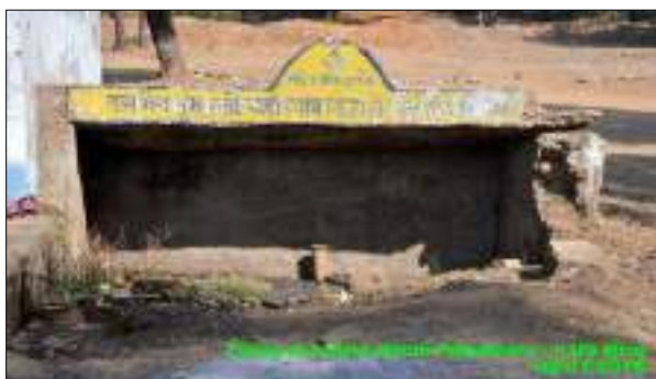
Before- Open incline entry prior to sealing
