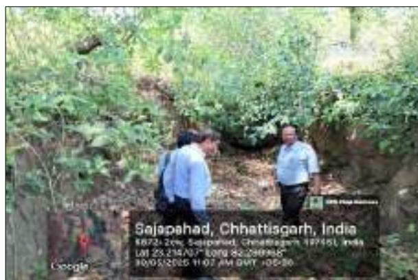
Before- Open mine entry prior to sealing
