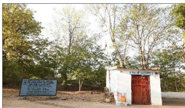
After-Incline entry sealed and secured
