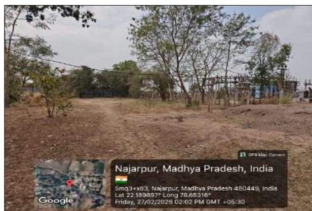
After- Cleared and Restored Site
