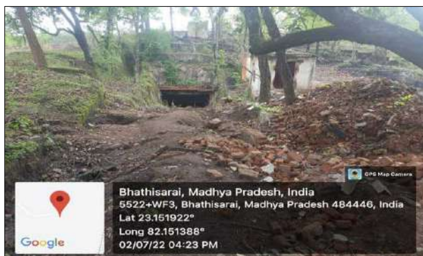
Before- Mine Entry Prior to Closure
