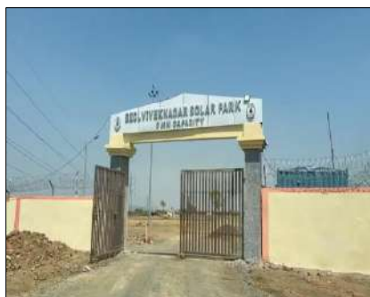
Eco-park on reclaimed land
