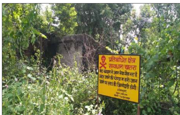
Before - Sealing of Entry
