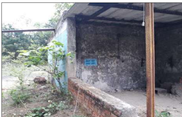
Before- Pre-Dismantling Condition
