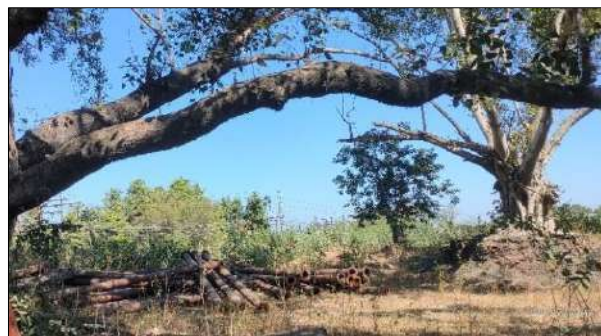
After- Cleared Land (Post-Dismantling)
