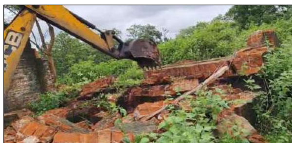
Before- Existing Structure (Fan Shaft)
