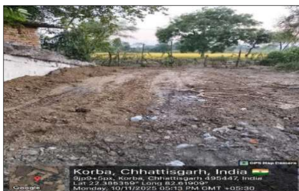
After- Sealed and Secured
