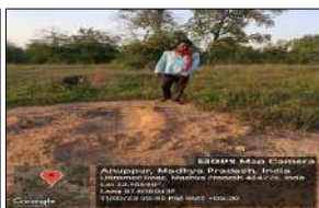
After-Pits Filled and Prepared for Plantation
