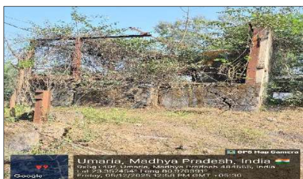
Before- Existing Structure (Pre-Dismantling)
