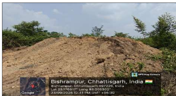
After- Secured and Sealed Incline
