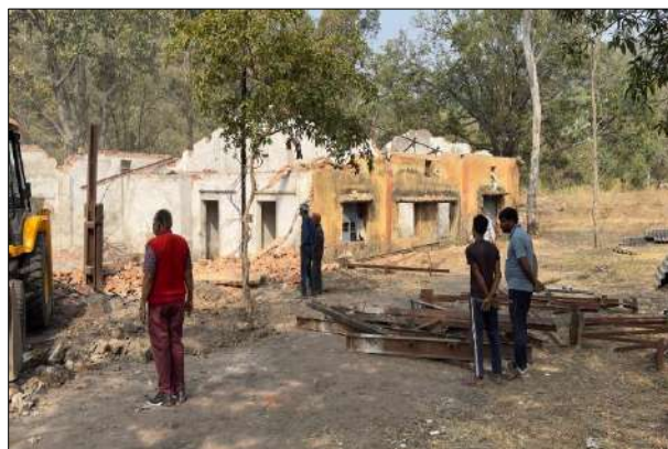
Before- Existing Structure (Pre-Dismantling)
