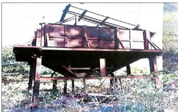
Before- Existing Structure (Pre-Dismantling)
