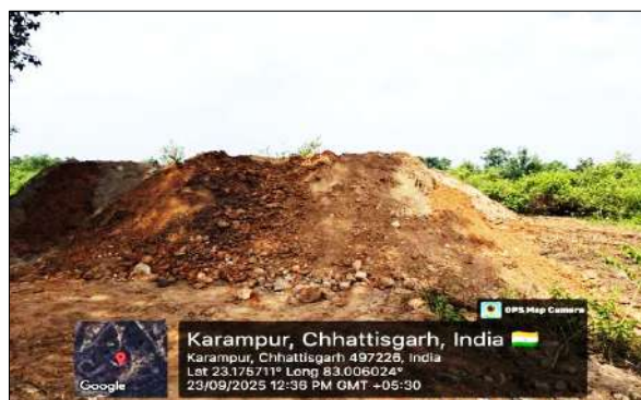
After- Sealed and Stabilized Entry
