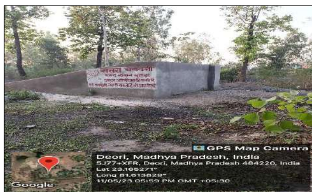
After-Sealed and secured
