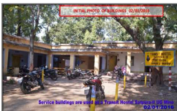
Before- Existing Structures
