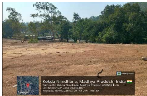
After- Cleared and Restored Site
