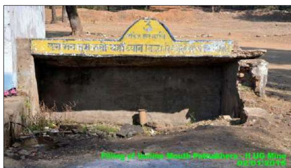
Before- Open incline entry prior to sealing
