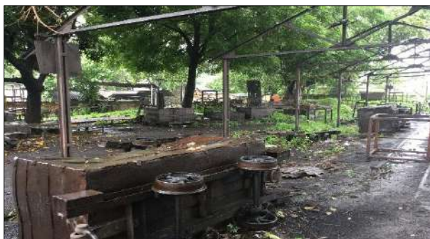
Before- Existing Structures (Pre-Dismantling)
