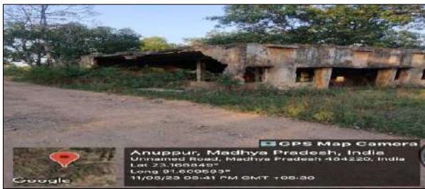
Before- Pre-Dismantling Condition
