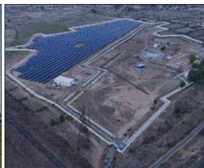
Aerial view- Operational Solar Plant
