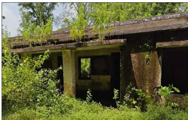
Before-Abandoned concrete structure
