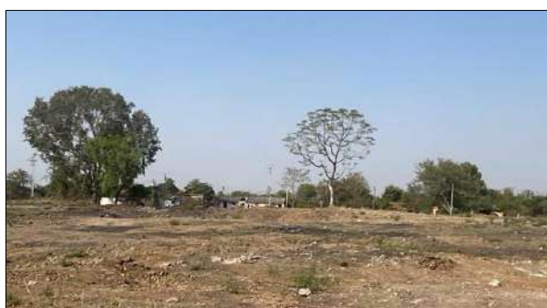
After- Mine entries Scientifically Sealed & Reclaimed
