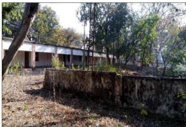
Before- Existing Infrastructure (Pre-Dismantling)
