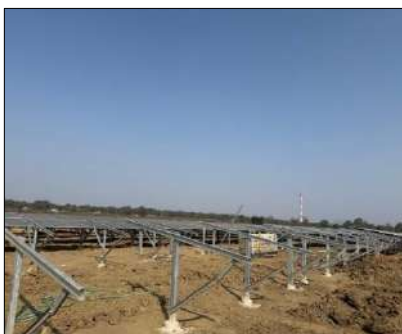
Solar Plant under installation
