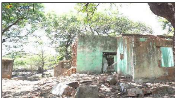
Before- Existing Structure (Pre-Dismantling)
