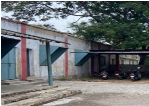
Before-Existing Building Structure
