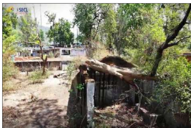
Before- Mine Entry Prior to Closure
