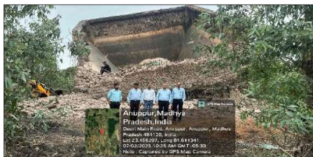
Before - Pre-Demolition Condition of Site
