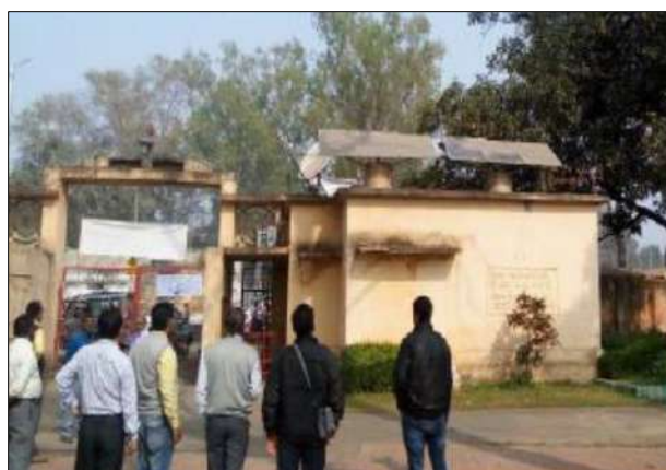
Before- Dismantling of Existing Structures
