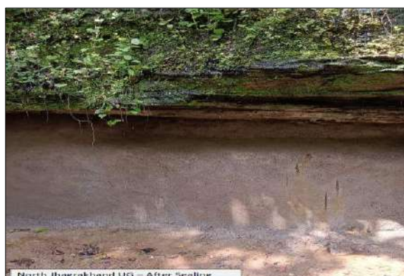
After- Secured and Sealed Incline
