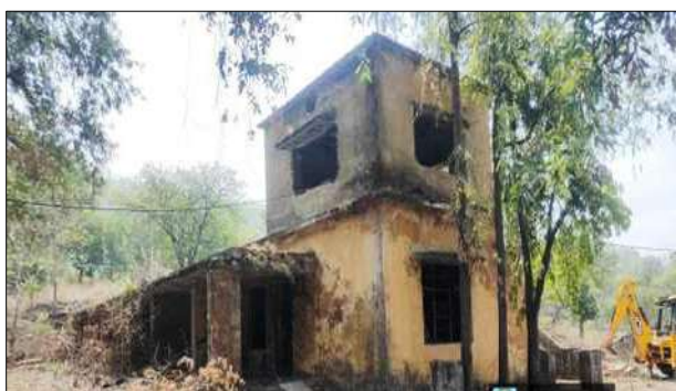
Before- Existing Structure (Pre-Dismantling)
