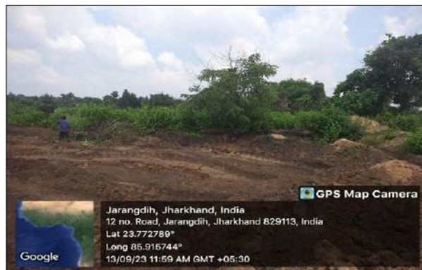
After- Site cleared and levelled for future utilization
