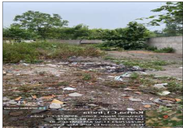
After- Site Cleared Following Demolition Activities
