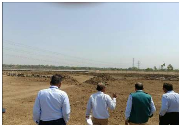
After-Site cleared for utilization
