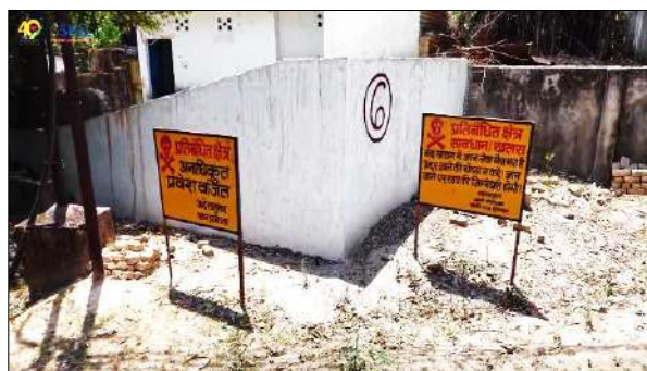
After- Secured and concrete sealed Incline
