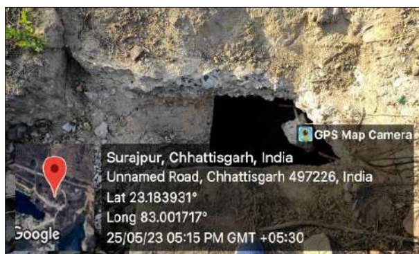
Before- Open Mine Entry (Pre-Closure)
