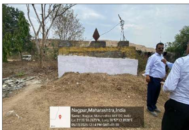
Before- Mine Incline Prior to Closure
