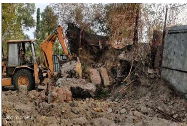
Before- Existing Structure (Pre-Dismantling)
