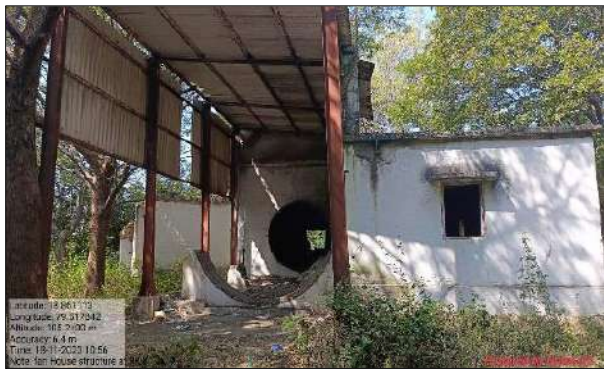
Before- Airshaft structure prior to dismantling
