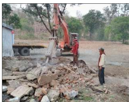
Before-Prior to dismantling
