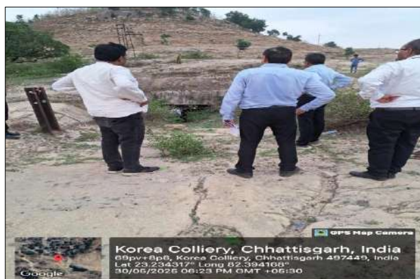
Before- Open Mine Entry (Pre-Closure)
